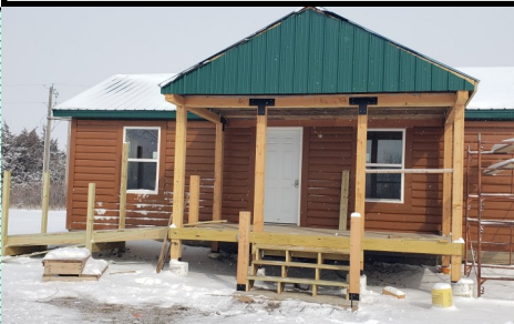
White Rock Cabin, In Progress
